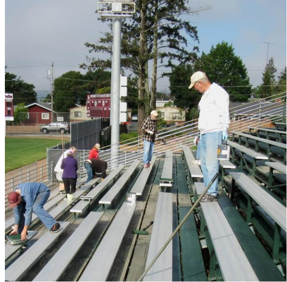
Dan inspecting the work
